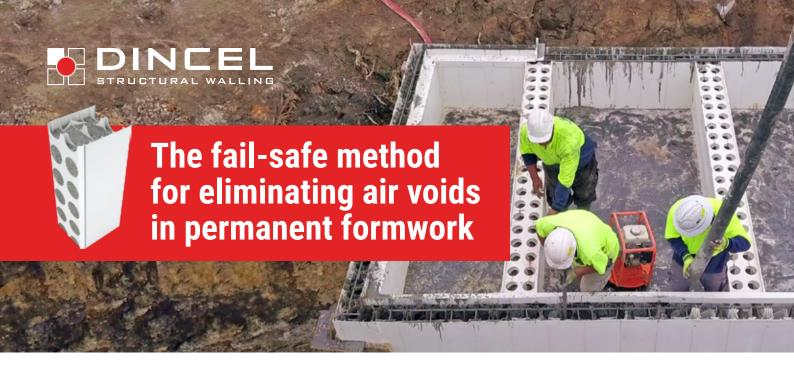
Designed to withstand the high pressures generated from the use of vibrators and high slump concrete, Dincel 275 ensures the elimination of air voids when the following is adopted:
