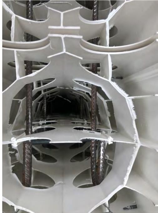
**Figure 5: Dintel panels with shear steel reinforcements (before pouring concrete)**
