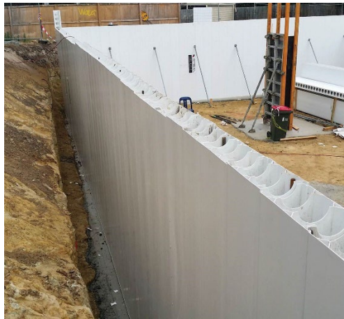
Figure 1 (Dincel PVC formwork and some steel reinforcing prior to concrete)
