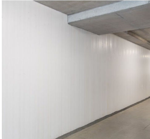
Figure 2 (Typical basement Dintel wall - no attachments)
