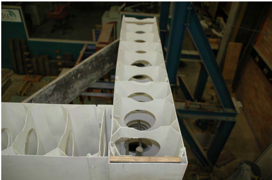
Fig 4.3 – Wall specimen ready for concrete pouring
