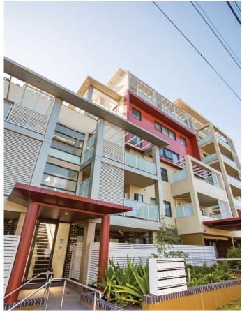
The Dincel Wall applications include 200 Dincel Wall for retaining walls, fire corridor walls, lift shaft walls and stair shaft walls. 110 Dincel Walls were adopted for all apartment inter-tenancy party and corridor walls and 200 Dincel Walls were adopted for all external facade walls.
