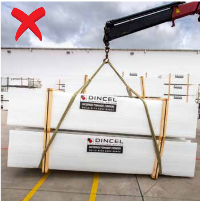
INCORRECT LIFTING (No lifting/spreader bar used)
