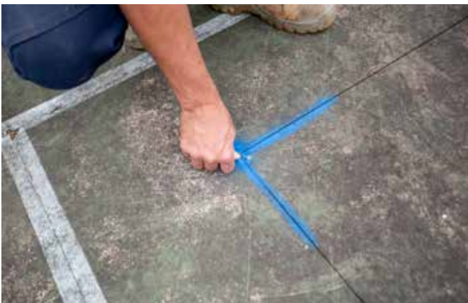
2: Use chalk line to mark out wall base location in accordance with the consultant drawings. Work off gridlines or surveyor marks for accurate placement.
