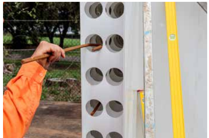
12: Place corner horizontal reinforcement into wall:
