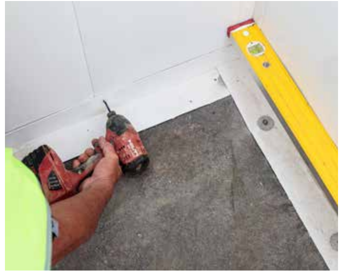
10: Screw fix bottom of panels into angle, ensuring that the corner assembly is square.
