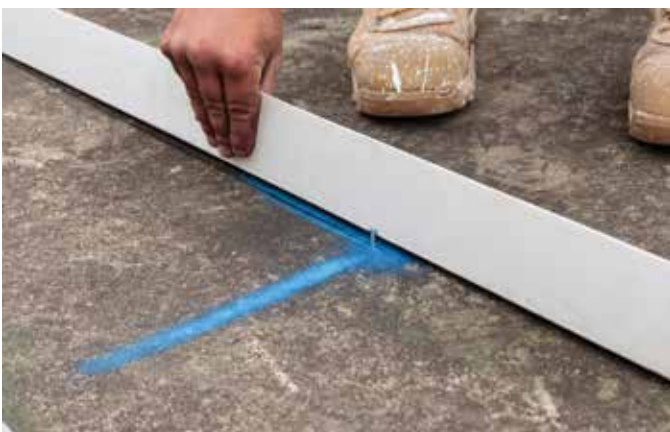
3: Place D-ANG50 PVC Angle along the chalk line mark. Place angles on one side only for conventional concrete or on both sides for self-compacting concrete.
