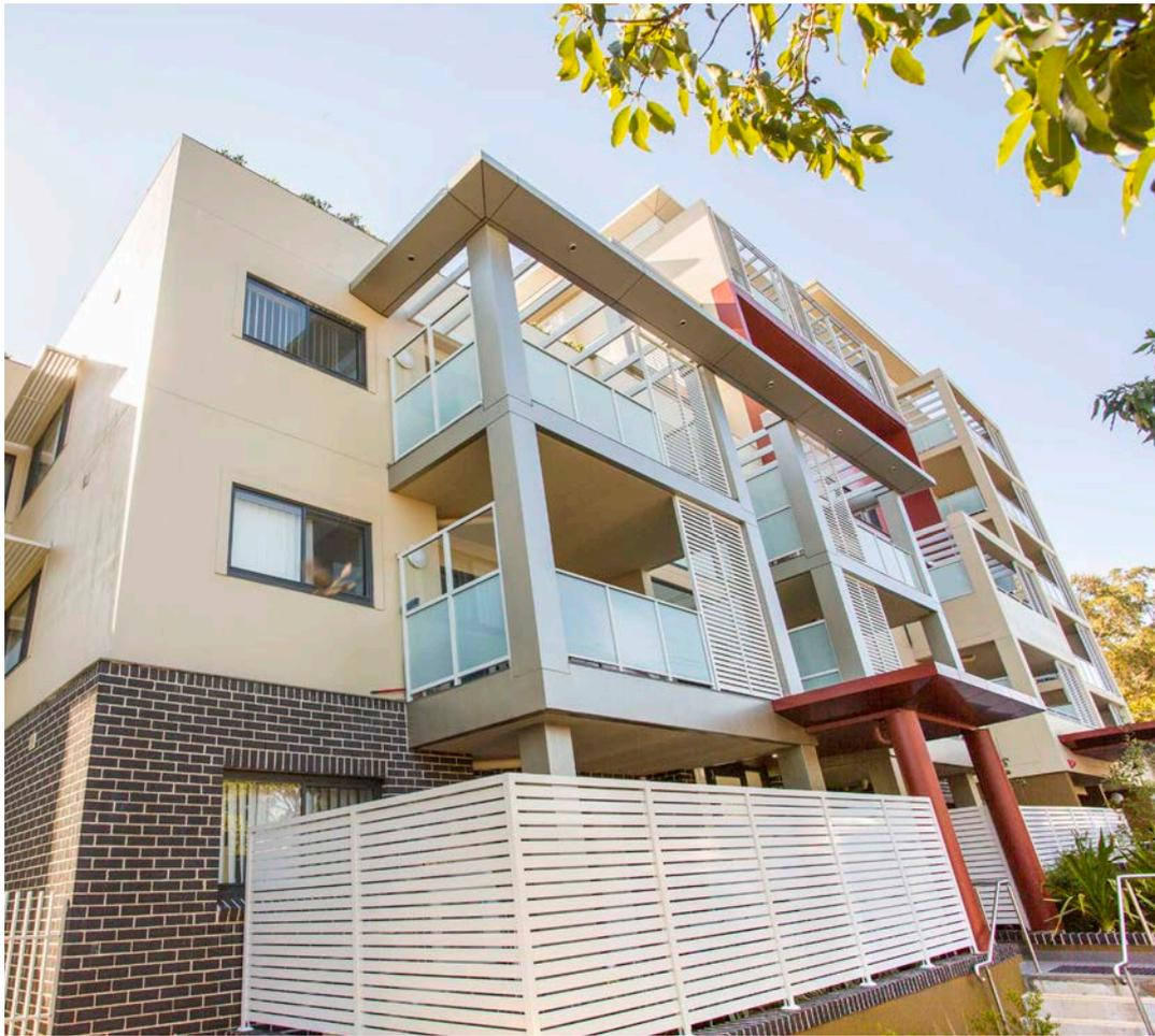
**“WE HAVE TAKEN ADVANTAGE OF UTILISING THE DINCEL LOAD-BEARING WALLING SYSTEM IN CONJUNCTION WITH CONVENTIONALLY-FORMED 150 TO 170MM THICK FLOOR, REINFORCED MESH SLABS.”**
