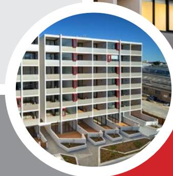
“The build used 200mm Dintel in the basement, lift, stair and service shafts and well as for deep beams, blade columns and façade walls. In other areas, 110mm Dintel walls were used for party walls in between apartments supporting 170mm thick slabs,” Mr Barakat said.
