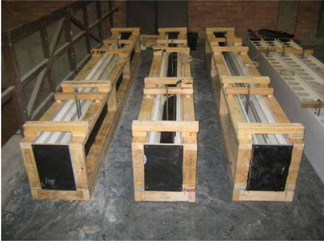
**Figure 15 – Completed formwork boxes**
