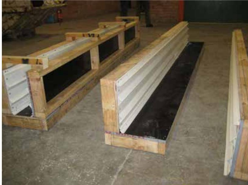
**Figure 6 – Formwork box construction**
