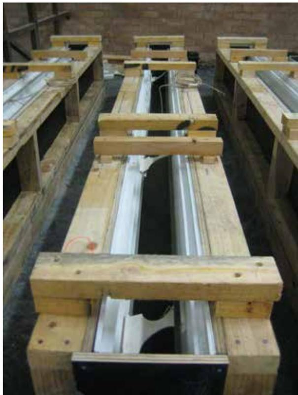
**Figure 12 – Reinforcement bar placement using pieces of P-J joiner module**
