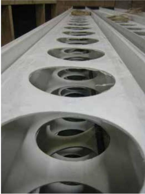
**Figure 22 – Reinforced Dintel samples ready for concrete pouring from closer angle**
