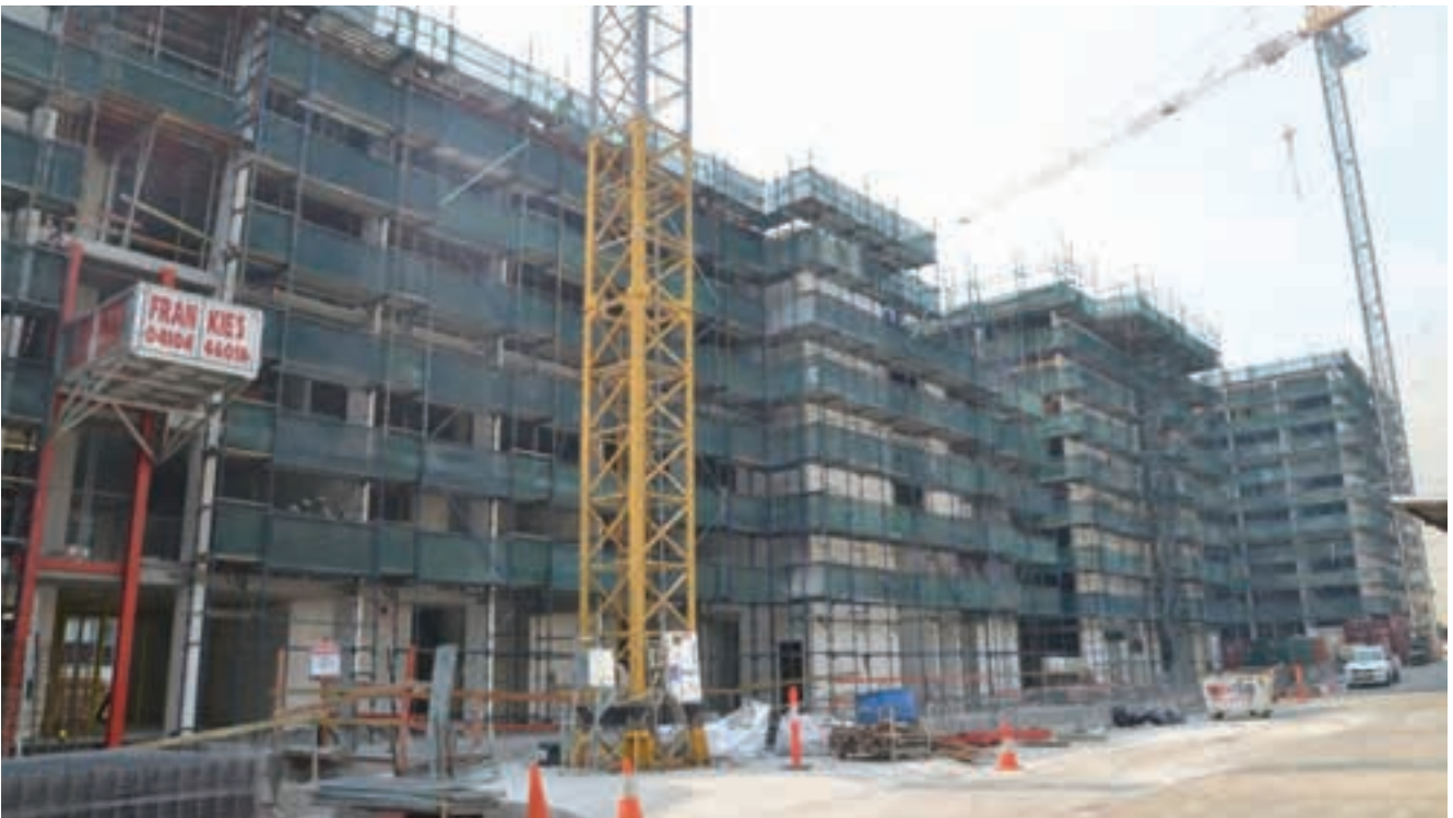
52 WEEKS CONSTRUCTION PROGRAM – REDUCED BY 26 WEEKS
